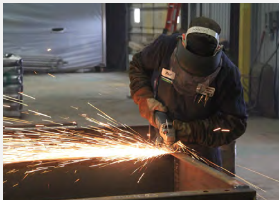
Above: Phil Jankoviak grinding at the North Shop
