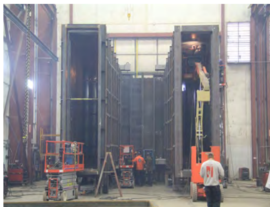
A recently completed module for the Consumers Energy Project.
