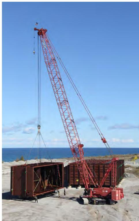
Moran Iron Works fabrication of baghouses is in mid stride, with 9 of 24 of these massive units truck shipped down the high wire corridor to our deep water port. Upon arrival they are test fitted together and inspected by a team of Certified Welding Inspectors (CWI).
