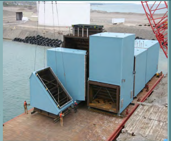
Barge loading of a Duct Work assembly May 2012
