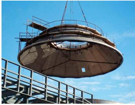
Absorber hood being lifted
