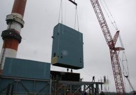
Babcock & Wilcox-Consumer's Energy Project units being lowered into place during installation
